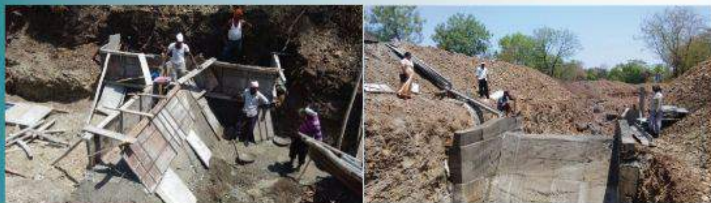
The construction of the third check weir constructed with the help of WRSSF and also the friends of Mr. Ronald D'Souza
